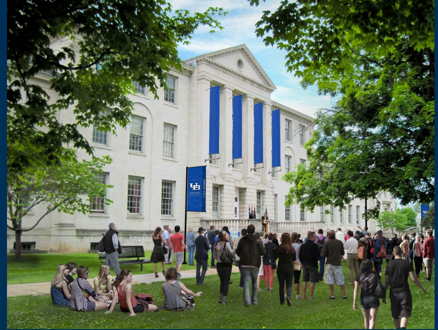
Parker Hall South Campus Status: Program Verification Phase $135M
